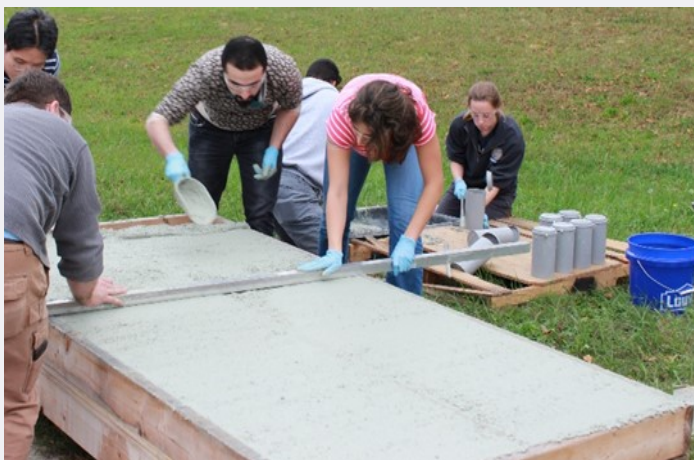
Caption: Latex Modified Concrete Overlay during the casting.
